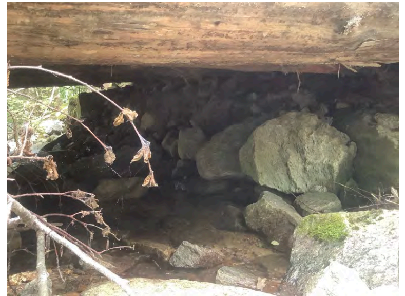
Right Bank Abutment when facing downstream
