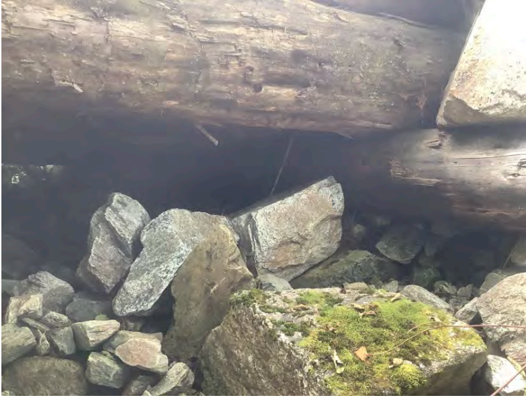
Left Bank Abutment when facing downstream
